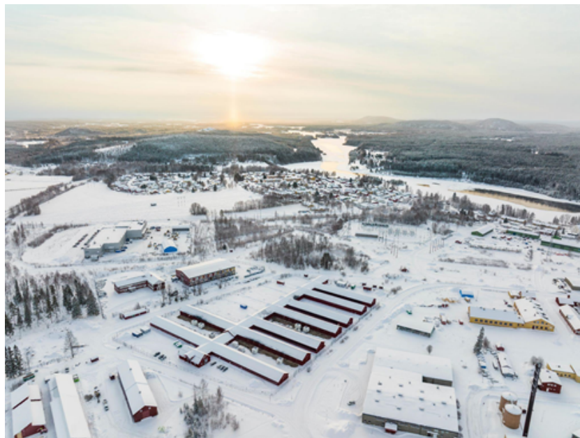
Figure 6: Hydro66 campus is 7000m2 and 40 MW installed capacity
